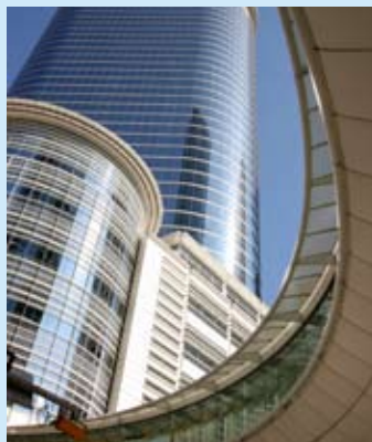
Chevron Offices Houston, Texas
